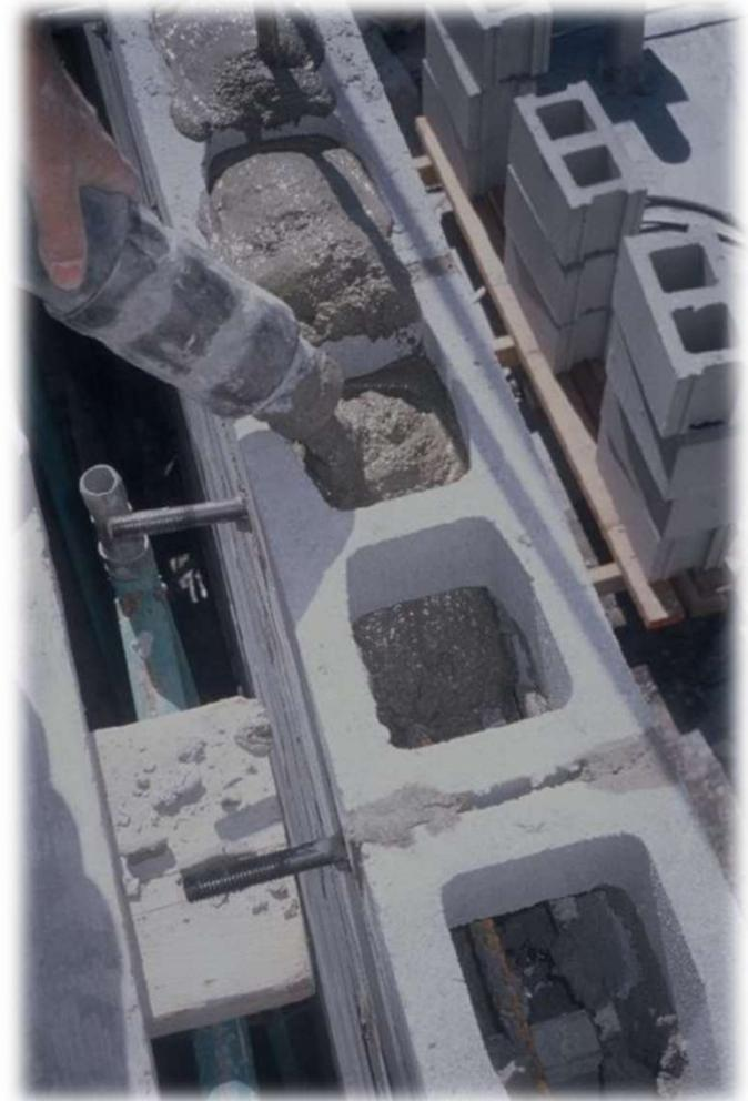
Grout is like micro-concrete: a mix of cement and sand (fine grout), and in some cases small-size aggregate (coarse grout)
