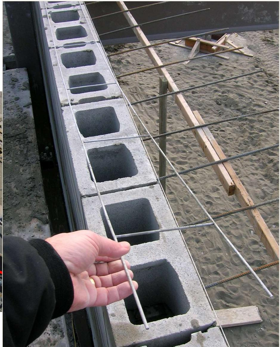
Joint (ladder) reinforcement
