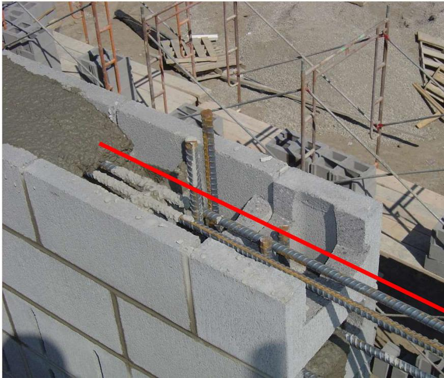
Bond beam reinforcement
