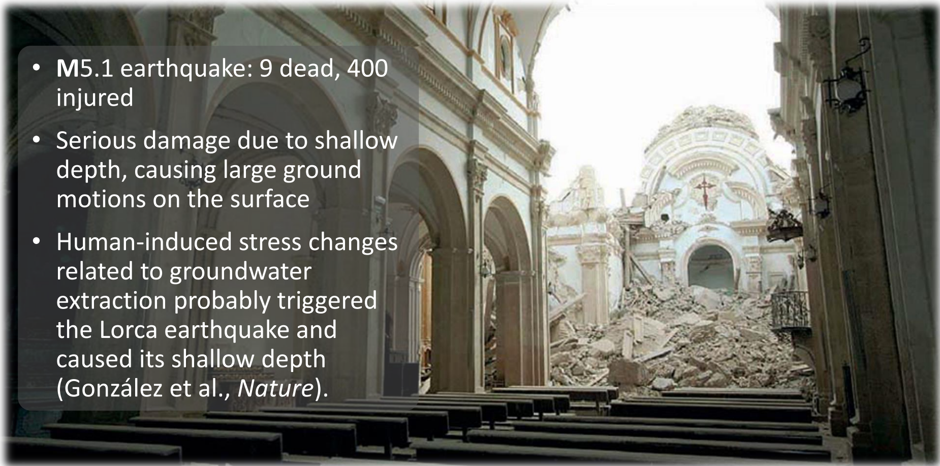
The Lorca Earthquake caused widespread damage, and destroyed the St. James church, pictured here. (Photo: Creative Commons)
