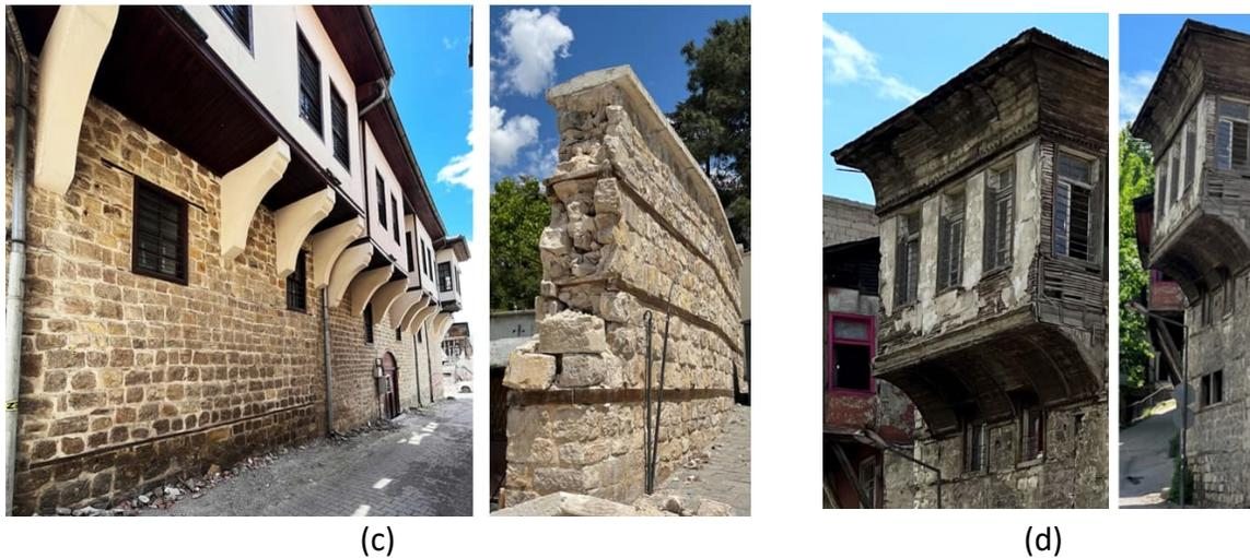
**Figure 7.6: Traditional building typologies (a) Timber frame with masonry infill, (b) Adobe building (Malatya) and (c) Timber laced masonry wall construction (Kahramanmaraş), (d) “Bagdadi” – short pieces of timber studs used for infill (Kahramanmaraş)**
