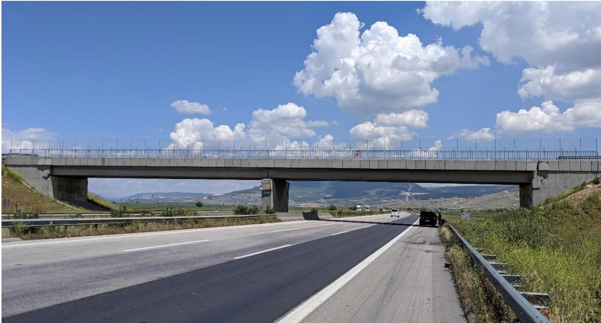
**Figure 8.1: Typical Highway Underpass**
