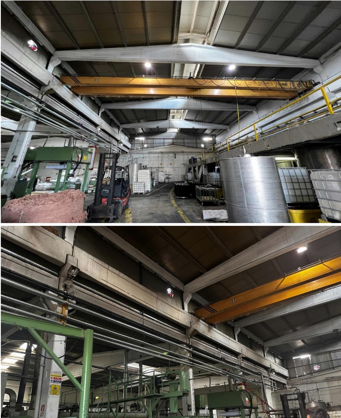
**Figure 6.38: Precast concrete frame industrial facility, Gaziantep [37.16311557, 37.29198872].**
