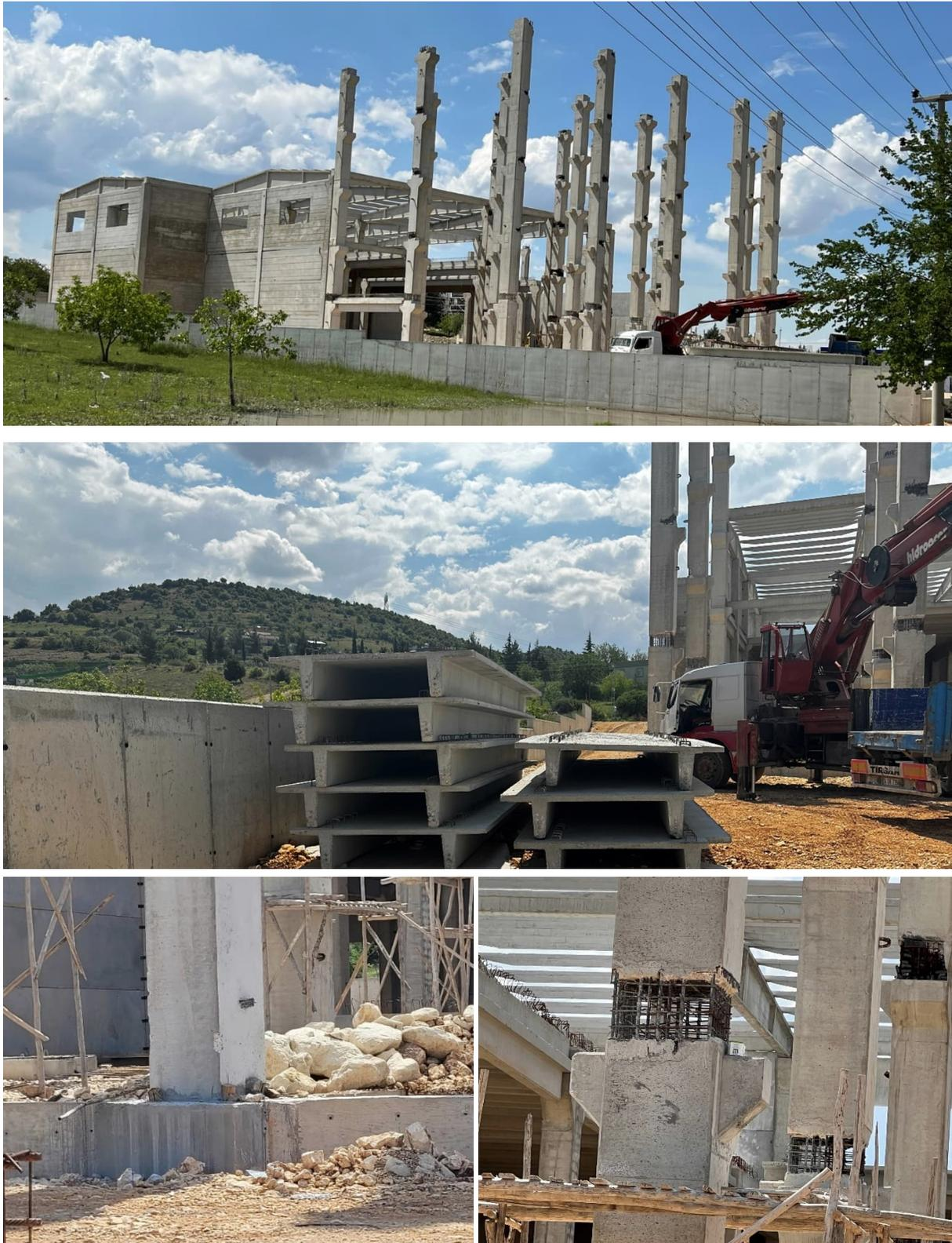
**Figure 6.43: Pre-cast concrete frame under construction, Aktoprak [37.18609275, 37.2723584].**
