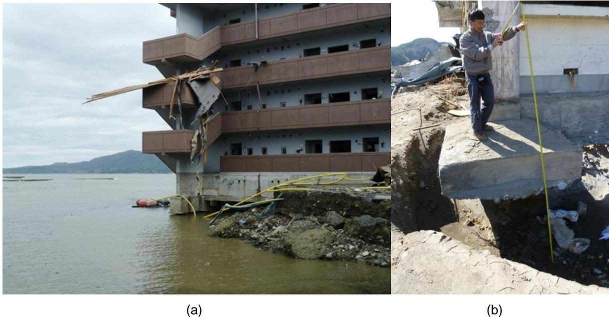
**Fig. 9 – (a) Scour due to return flow around apartment building in Minamisanriku; (b) Foundation scour at the corner of reinforced concrete building in Taro (Chock et al., 2012)**
