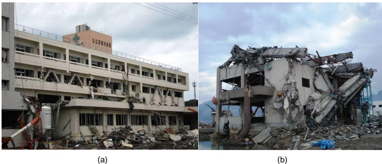
**Fig. 7 – (a) Minamisanriku Hospital – RC building withstood tsunami loading (Chock et al., 2012); (b) RC building with collapsed steel trusses top floor**
