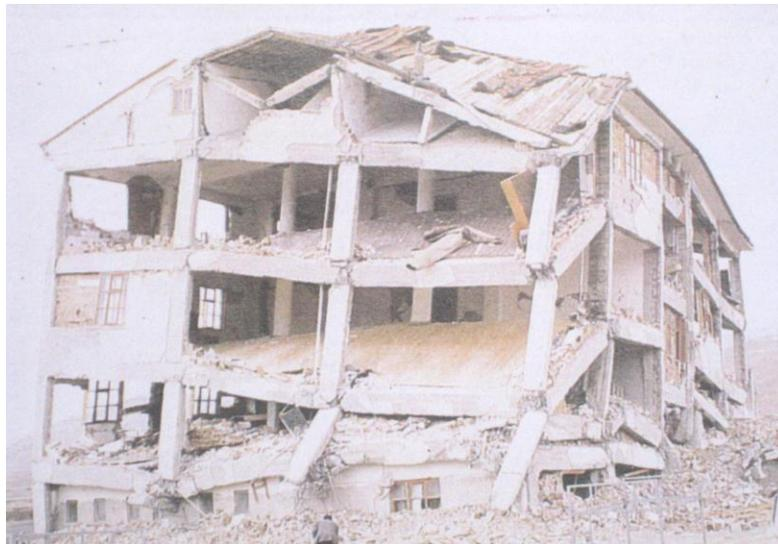
**Fig. 2 – Joint Failure and Partial Building Collapse in the March 13, 1992, Erzincan, Turkey Earthquake, (Photo Credit, Zahertar)**
