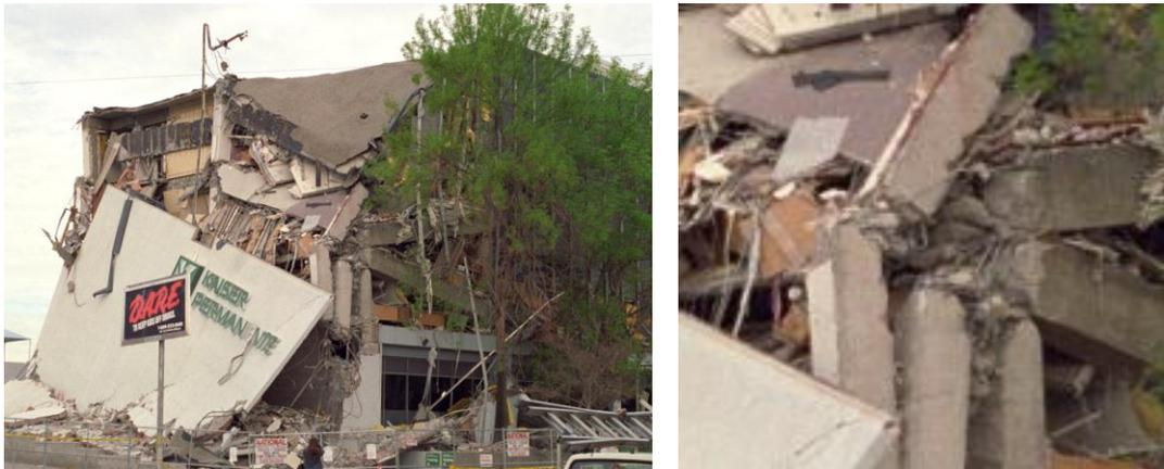
**Fig. 1 – Structure Collapse due to Failure of Deficient Beam-column Joints, Kaiser Permanente Building, Northridge Earthquake, 1994 (Photo Credit, G. Edstrom)**
