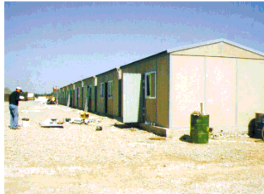
Fig. 18. Serdivan — Prefabricated “temporary” housing under construction.
