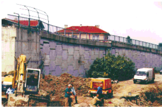
Fig. 4. Arifiye — Reinforced earth abutment at TEM overpass.
