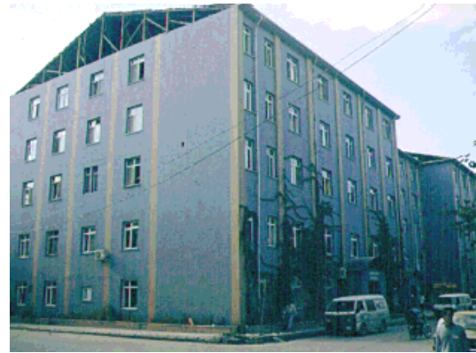
Fig. 10. Sakaraya — Maternity hospital gable-end.
