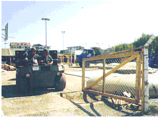
Fig. 16. Serdivan — 15 000-L rubber bladder temporary water reservoir.
