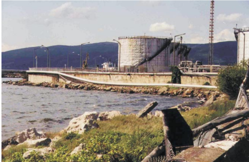
Fig. 29. Dislocated pipes along the seashore.
