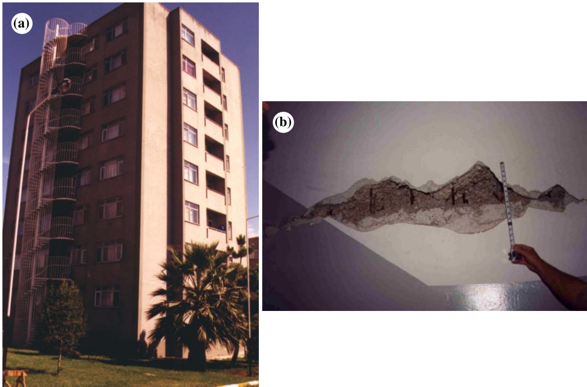
Fig. 12. Frame wall building in Izmit without significant damage: (a) exterior view and (b) structural wall with concrete placement problem.
