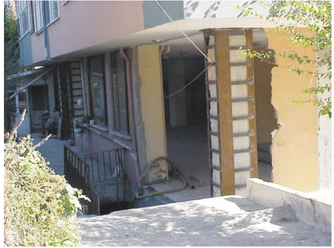
Fig. 37. Shear failure of ground-storey column.
