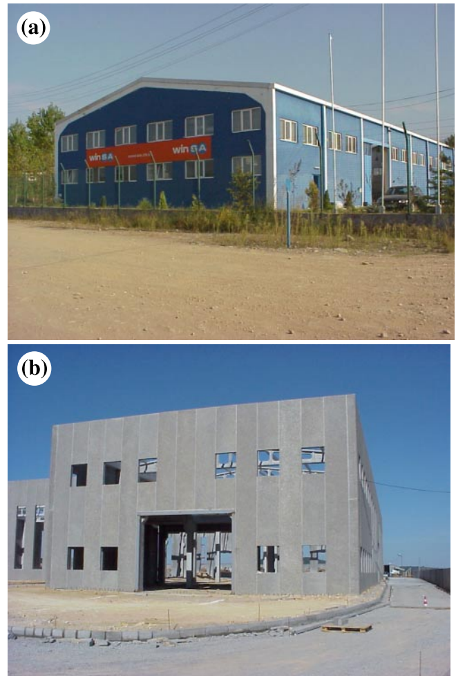
Fig. 20. Examples of precast structures that performed well.
