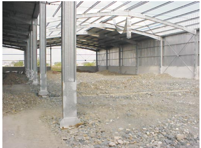
Fig. 21. Cold-formed steel structure.
