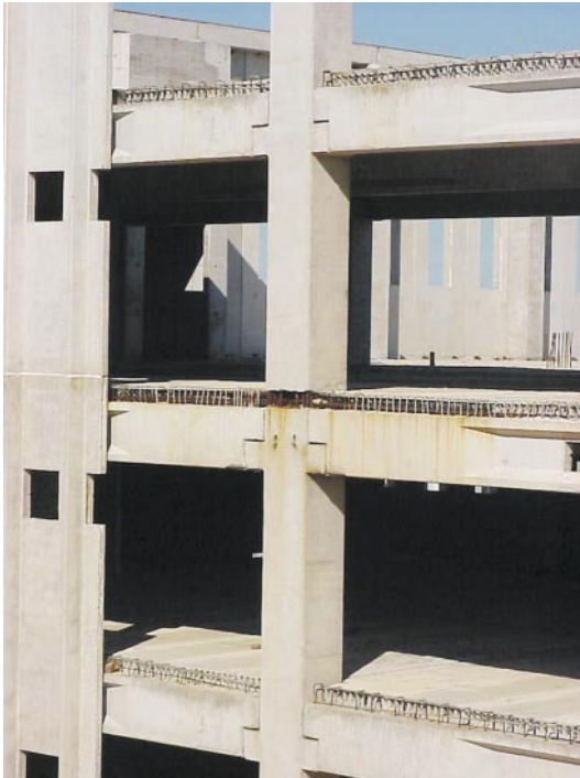
Fig. 35. Precast concrete structure under construction.
