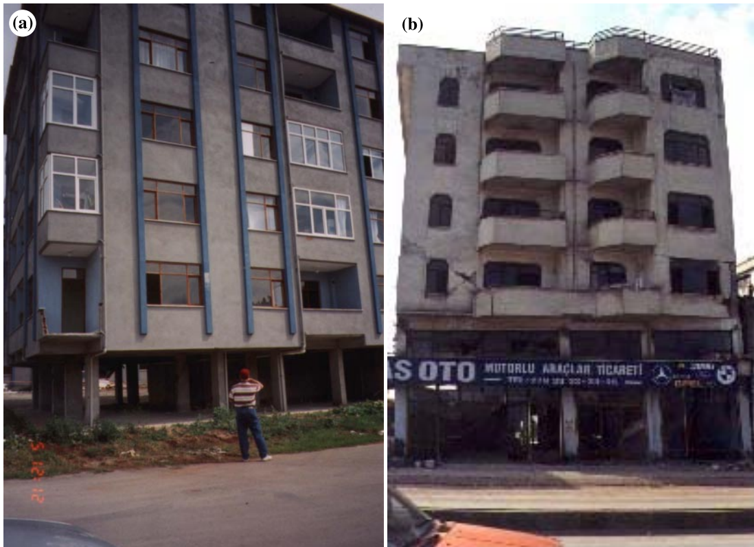
Fig. 3. Examples of soft storey reinforced concrete buildings.
