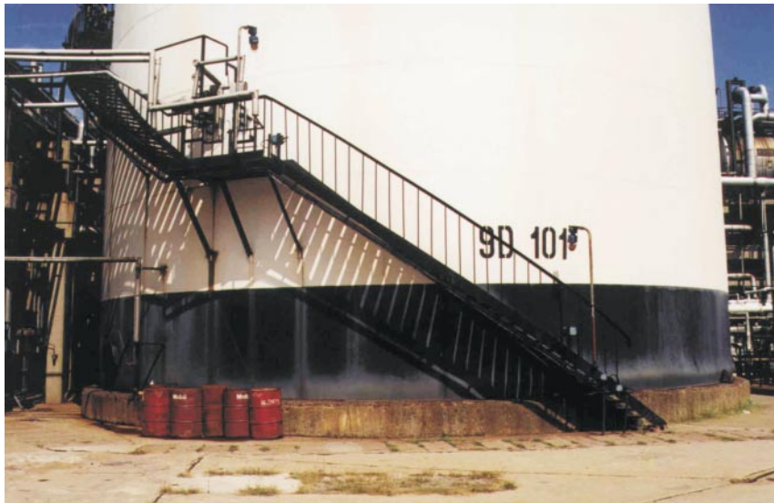
Fig. 28. Close-up view of the elephant foot type buckling.
