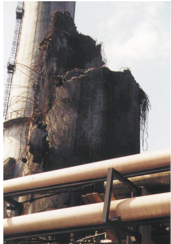
Fig. 23. Chimney failure at Tupras Oil Refinery.
