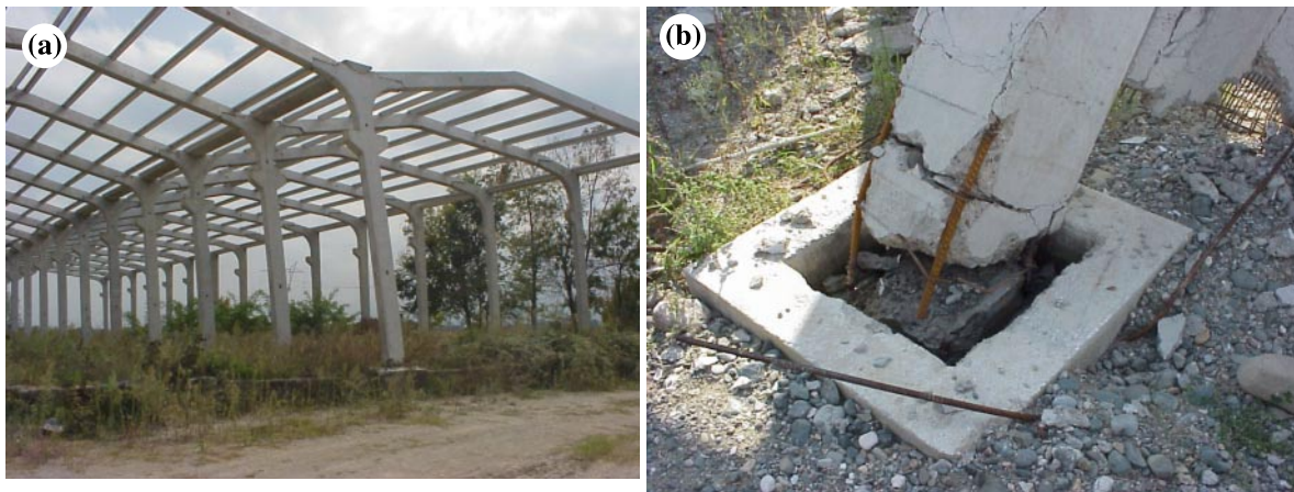
Fig. 14. Typical precast industrial building: (a) frame with short cantilevers supporting cranked beam and (b) column socket at base.
