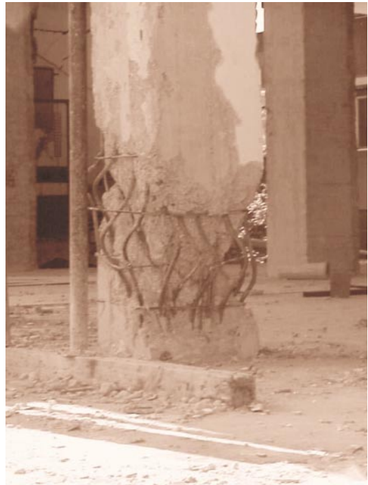
Fig. 37. Shear failure of ground-storey column.
