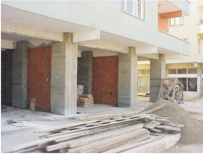
Fig. 38. Concrete columns after retrofit.
