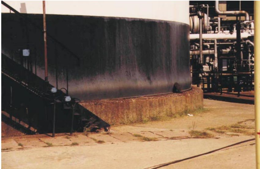
Fig. 28. Close-up view of the elephant foot type buckling.
