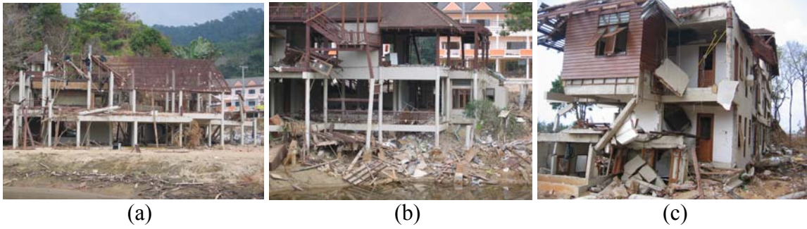
Fig. 7 Structural damage in Nai Thon Beach due to tsunami waves
