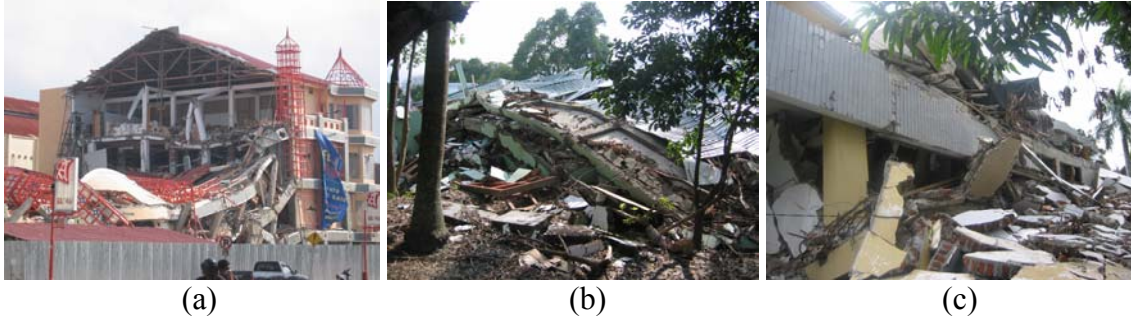
Fig. 12 Earthquake damage in Banda Aceh, Indonesia
