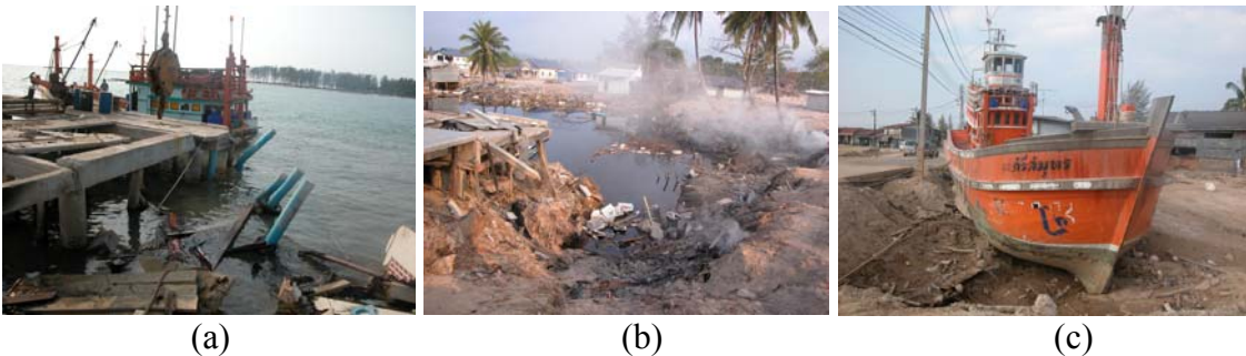
Fig. 9 Damage to Khao Lak harbor town
