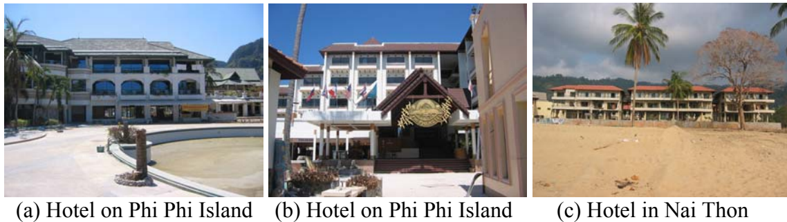
Fig. 19 Engineered concrete buildings survived tsunami forces without structural damage
