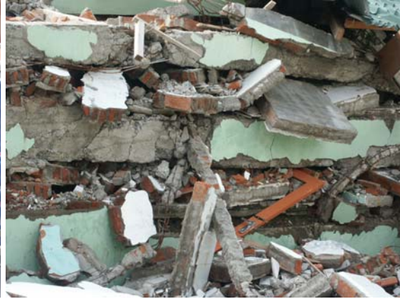
(b) Office building in Banda Aceh
