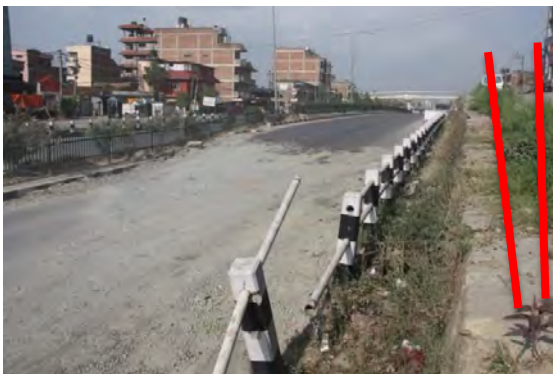
Figure 3.6: Road slump (after repair)
