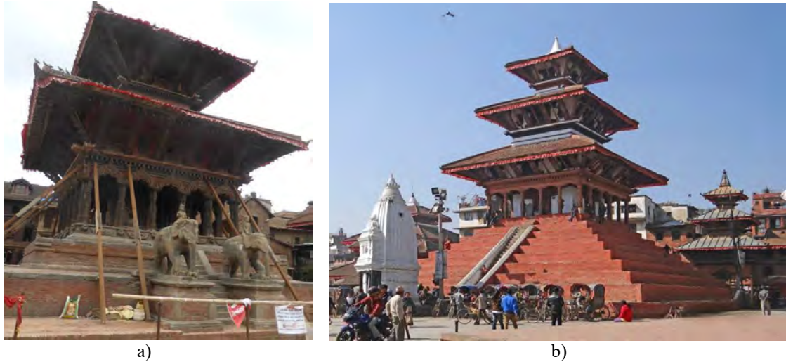
Figure 8.18: Multi-tiered Hindu temples in Nepal: a) two-tiered Vishwanath temple, Patan after the 2015 earthquake (S. Brzev) and b) three-tiered Maju Deval Temple, Kathmandu in 2013--the temple collapsed in the 2015 earthquake (Wikimedia 2013).
