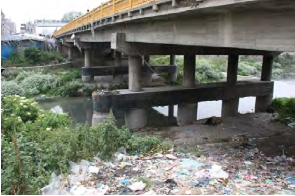
Figure 3.4: Substructure view June 11, 2015
