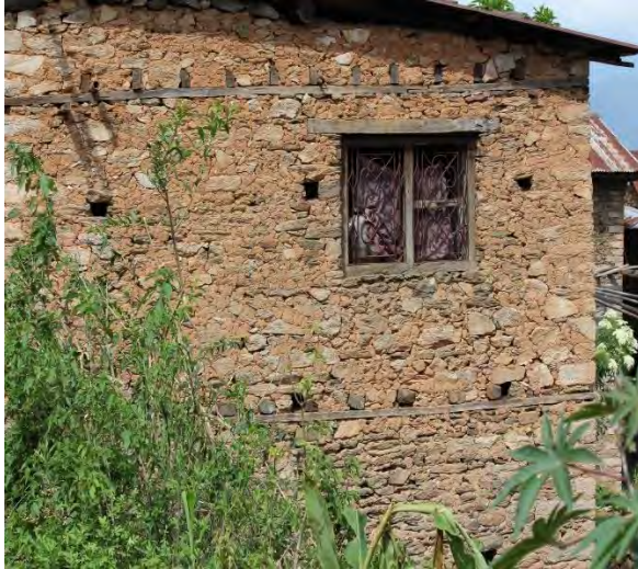
a) Details of timber bands
