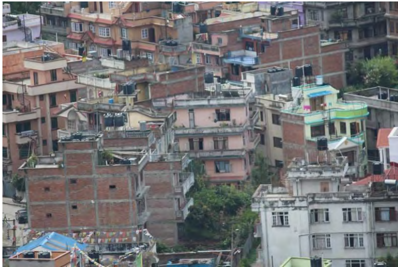
Figure 5.1: Skyline of Kathmandu showing predominantly low-rise RC construction with masonry infills (Photo: Bishnu Pandey)
