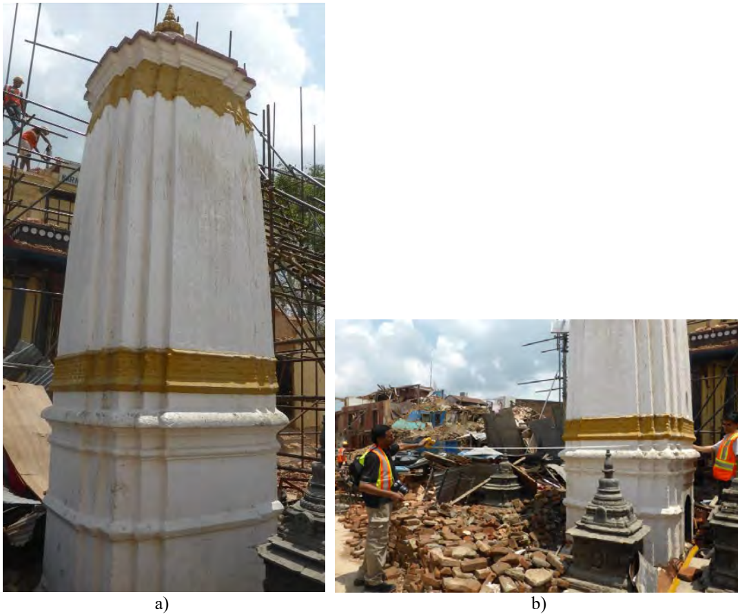
Figure 8.12: A sikhara-type shrine close to Pratappur temple: a) an exterior view, and b) CAEE team members Upul Atukorala and Bishnu Pandey taking field measurements of the shrine (S. Brzev).
