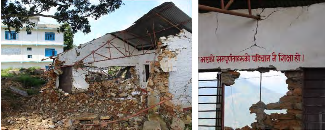
Figure 7.10: Complete collapse of stone masonry teaching resource centre building with concrete bands
