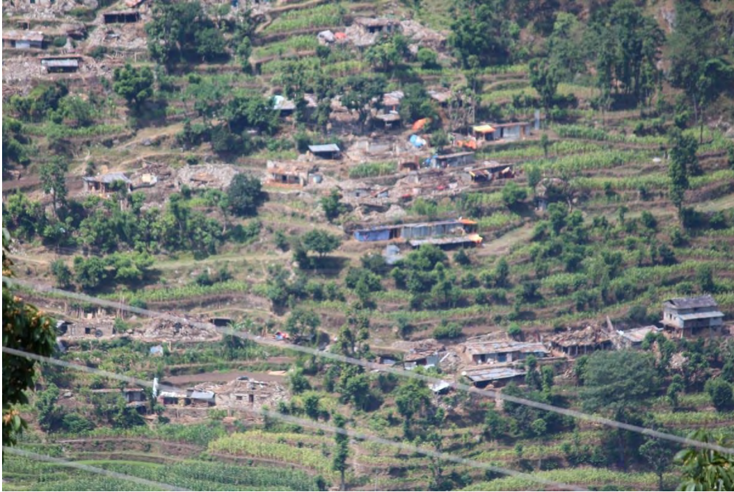
Figure 1.1: Extensive damage of rural stone masonry housing in Sindhupalchowk District (Photo: B. Pandey)
