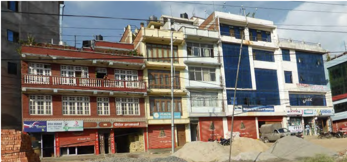
Figure 5.2: RC buildings with open storefront typical for Kathmandu and other urban and suburban centres in Nepal (Photo: Svetlana Brzev)
