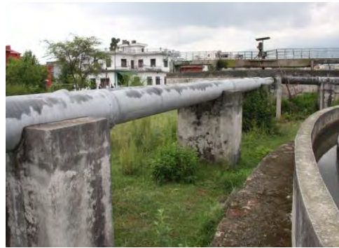
Figure 3.17: Connecting pipelines June 14, 2015
