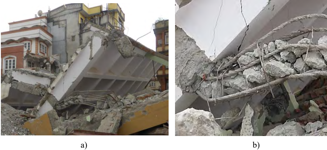
Figure 5.6: A collapsed 5-storey building at Khulesor, Kathmandu: a) ground floor level and b) detailing of column reinforcement (photos: Svetlana Brzev)
