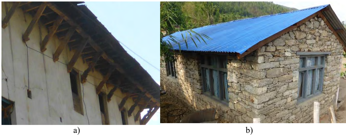
Figure 6.4: Typical roofs: a) traditional wooden roof and b) CGI sheet roof (Photos: S. Brzev)
