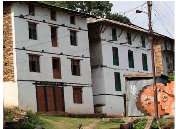
d) A four-storey stone masonry house with floor bands remained undamaged in the earthquake (Dolakha District).
