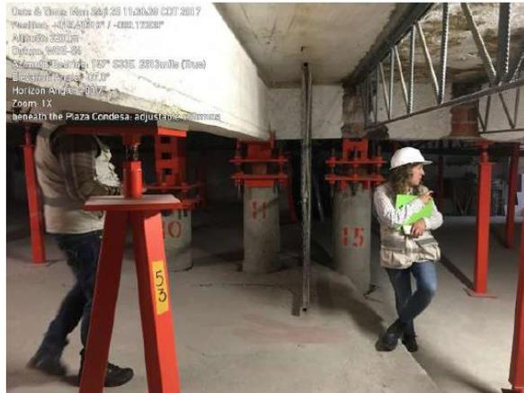
Fig. 16 End-bearing control piles supporting the La Plaza Condesa building (GEER 2018)
