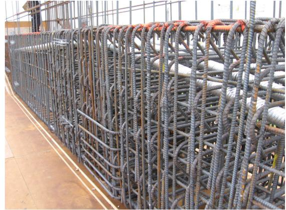
Figure 8. Pin zone reinforcement.
