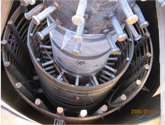
Figure 7. Pin inside column.
