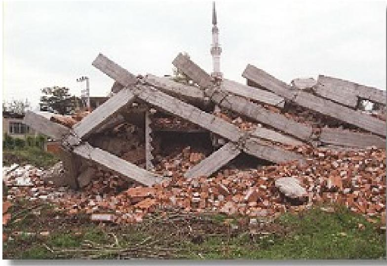
Figure 1. Total pancake collapse of a building because of inadequate design at the beam-column joints during the Kocaeli earthquake, Turkey, August 17, 1999, Magnitude 7.4.
