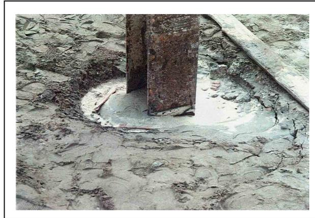
Figure 2. Soil subsidence around pile number 1.
