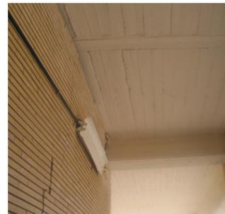
Out of frame walls, west side, middle floor, with maximum drift ratio of 0.9%
