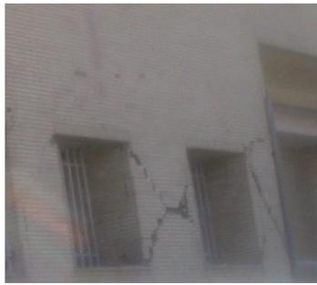
Failure of the infill wall, north side, in the middle floor, with corresponding maximum drift ratio of 0.9% from the analysis
