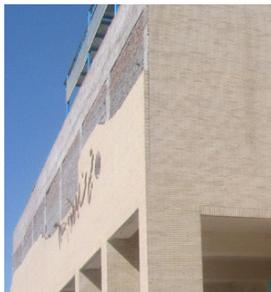
Failure of the infill wall south side top story, with max. drift ratio of 0.15%, however the crash was due to the torsion of the top beam, next to a bay of 13.2 m, with a rotational angle of 0.4%
