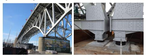
Figure 3. Granville Bridge: (a) elevation view, (b) replacement isolation bearings
