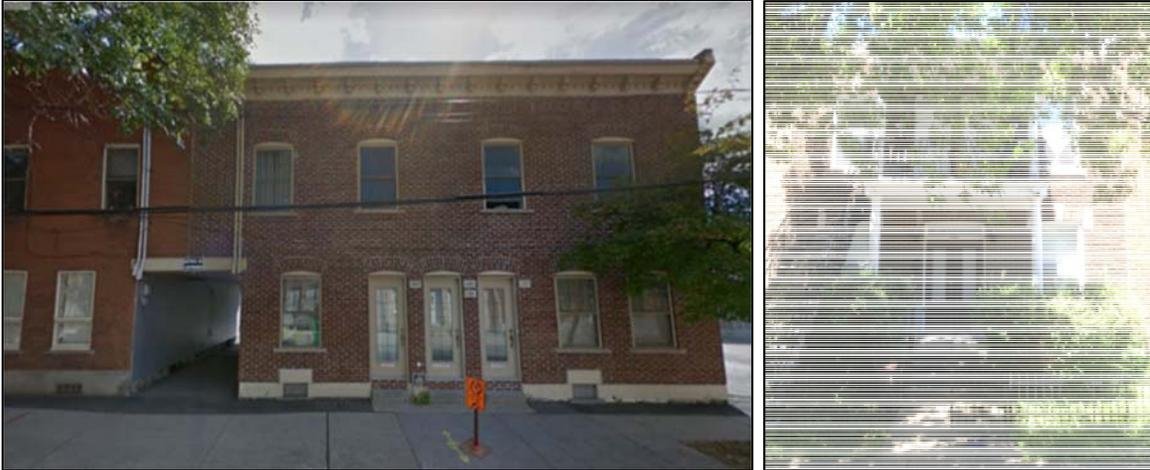
Figure 6 : Typical URM-B2 houses with spanning direction of the floor parallel to the street: (a) with carriage entrance located in South-West of Montreal, (b) with front staircase in Rosemont Petite-Patrie.
