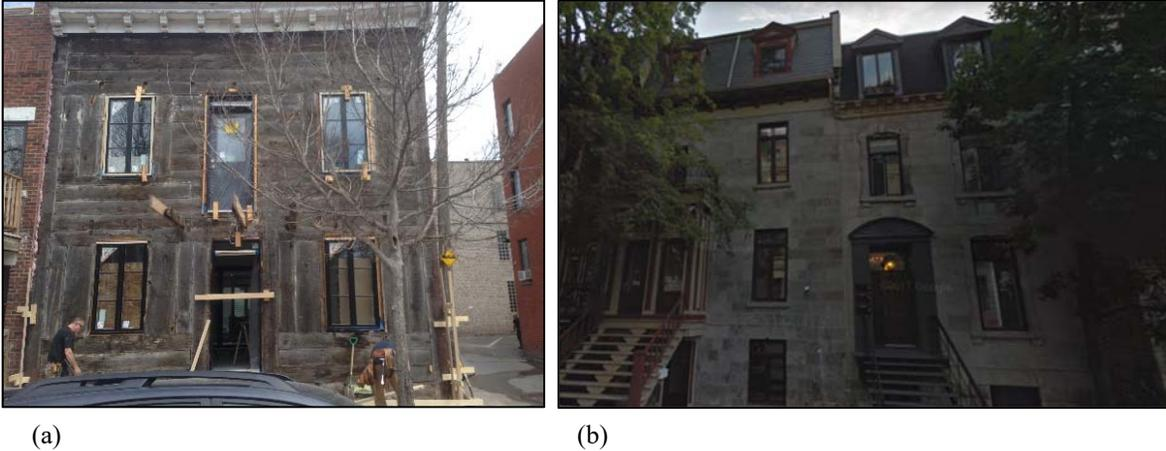
Figure 5: Typical URM-B2 houses: (a) timber plank wall, (b) 1865-1880 with floor system supported on the timber plank wall.
