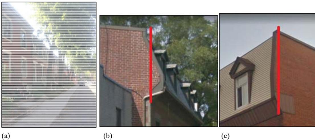
Figure 2: Typical URM-B1 houses: (a) in Westmount, (b) with real mansard roof, (c) with false mansard roof.
