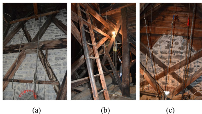
Figure 8. Examples of the structure of the bell tower at the level of connection with the façade: (a) the timber structure of the bell tower is attached to the façade masonry wall, (b) the structure of the roof intersects with that of the bell tower, (c) the timber structure of the bell tower starts inside the masonry of the façade.
