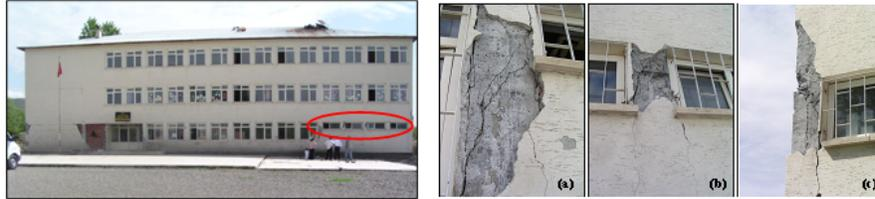
Figure 8. A three-story RC moment-frame template school in Bingöl after 5/1/2003 earthquake.
