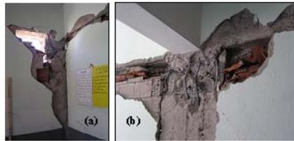
Figure 10. Typical captive column failures observed in (a) exterior and (b) interior columns restrained by full-bay masonry infill walls.
