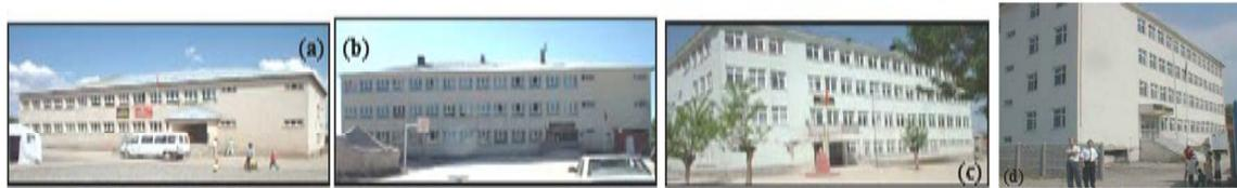
Figure 2. Typical RC school buildings with template floor plans. (a), (b), (c): structures with moment- frame system; (d) with dual system (i.e., moment-frames and shear walls).
