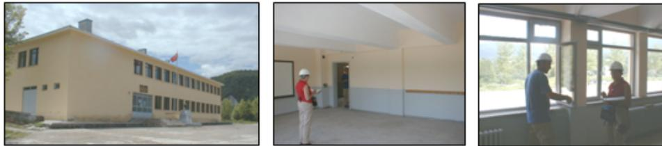
Figure 5. A two-story template RC dual system school building in Kaynasli near Düzce. No structural or non-structural damage during 8/17/1999 and 11/12/1999 earthquakes.
