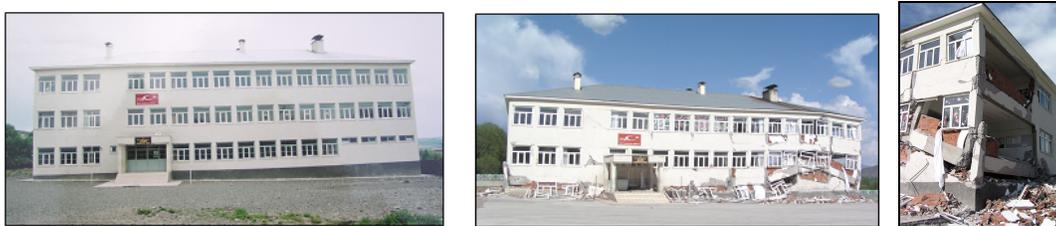
Figure 7. A three-story RC moment-frame template school building with captive columns in Bingöl before and after the 5/1/2003 Bingöl earthquake.
