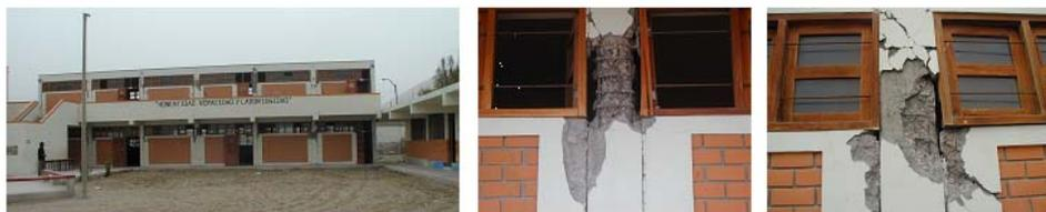
Figure 14. A template school building in Arequipa designed per the 1977 code after the 2001 Atico earthquake. center: a ground story column; right: a second story column. (Photo credit: Eduardo A. Fierro -BFP Engineers, Inc.-Bertero-Fierro-Perry.)
