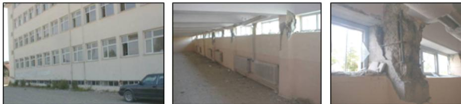
Figure 6. View of a dual system RC template school building in Düzce after the 12 November 1999 Düzce earthquake. The captive exterior columns in the basement failed.
