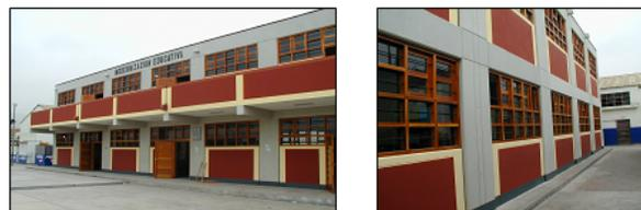
Figure 15. Views of a RC template school in Arequipa built per the 1997 Peruvian seismic code, seen after the 6/23/2001 Atico earthquake. No structural or nonstructural damage. (Photo credit: Eduardo A. Fierro - BFP Engineers, Inc.-Bertero-Fierro-Perry.)
