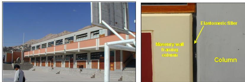
Figure 12. A school building in Peru built according to the template plan per the 1997 seismic code. Separation between the structural column and non-structural perimeter wall. (Photo credit: Eduardo A. Fierro - BFP Engineers, Inc.-Bertero-Fierro-Perry.)
