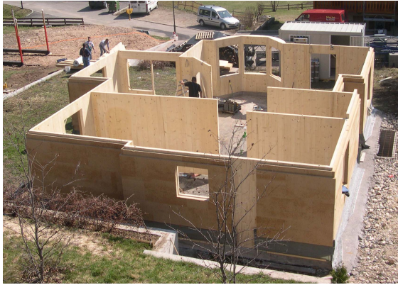
Figure 1. Typical X-lam building (Photo Rasom wood technology)
