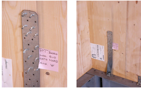
Figure 13. Hold-down failure after Nocera Umbra 1.2g
