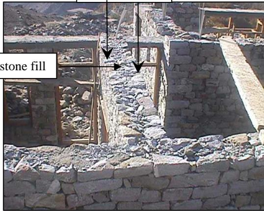
Figure 1: Typical Stone masonry building with two Wythes
