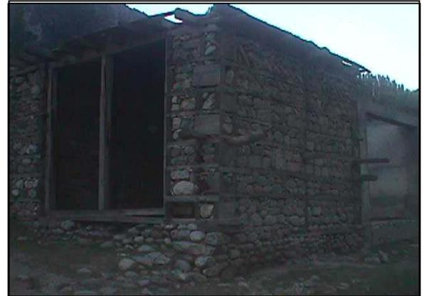
Figure 2 : Use of horizontal and vertical timber elements in stone masonry
