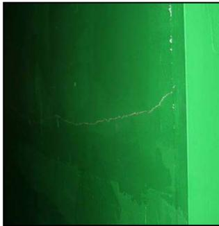
(q) Crack along partition wall
