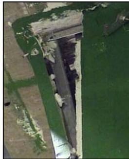
(b) Damage of corner beads/boundary studs
