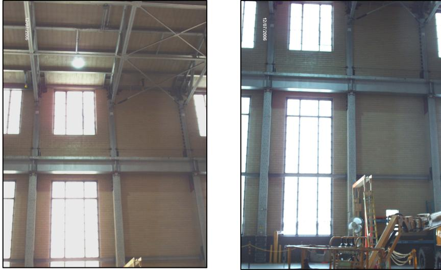
Figure 3. Part of the structure selected for ambient vibration measurements (frames 86 -88, middle of the powerhouse).
