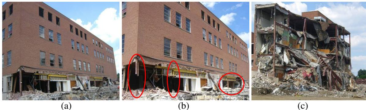
Figure 1. Before and After Removal of Four First-Story Columns of the Ohio Union Building
