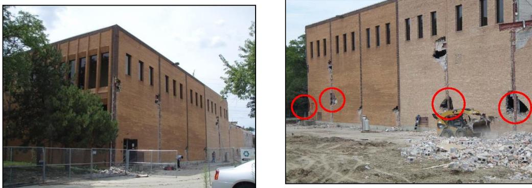
Figure 2. Before and After Removal of Four First-Story Columns of the BLCC Building
