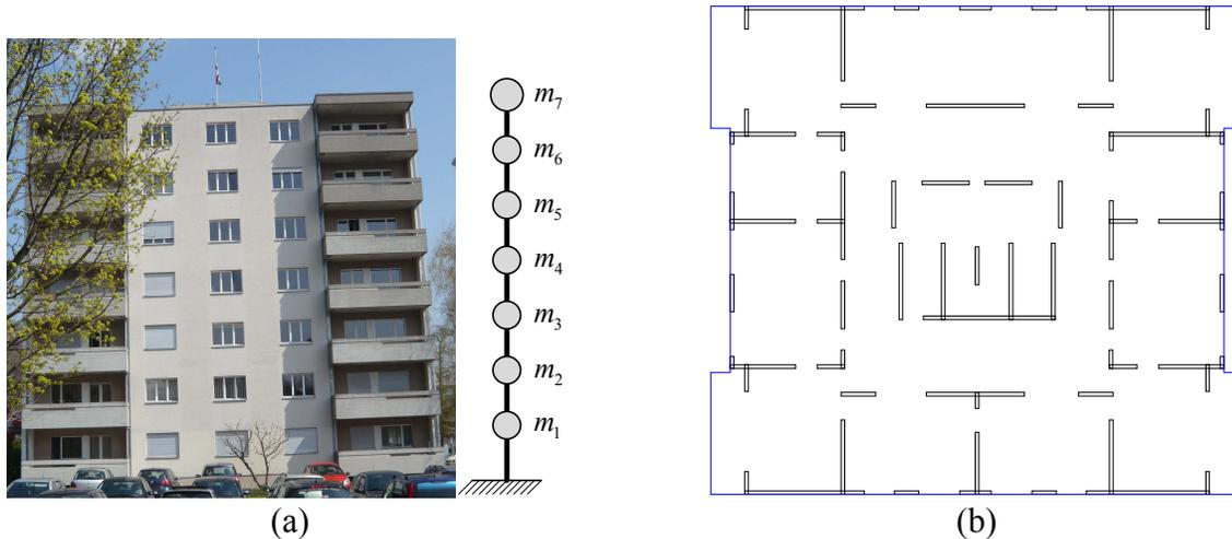
Figure 2. The 7-storey URM building in Delémont. (a) Picture of the structure and the corresponding beam model. (b) Plan (20[m]x20[m]) showing the different URM walls.
