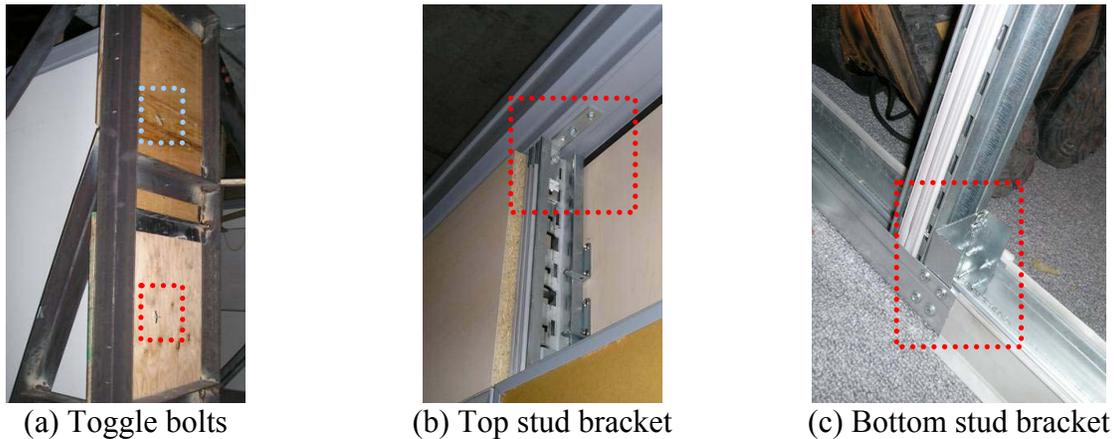
Figure 7. Joint reinforcement details in MOP-2R
