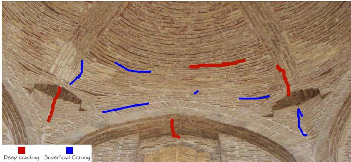
Fig. 7. Cracking pattern on the roof of Ivan
