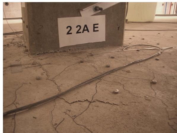
Figure 10. Vertical slab separations before limiting drift condition.
