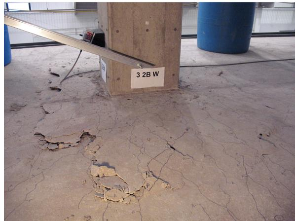
Figure 7. Slab column connection failure.
