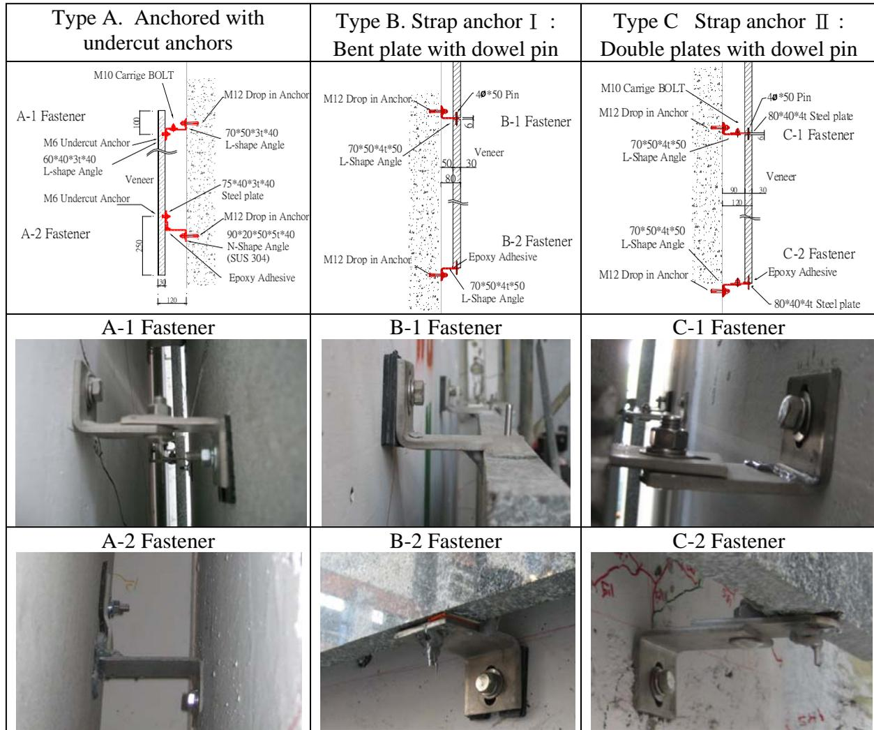
Figure 6. Details of Exterior Veneers (unit: mm)
