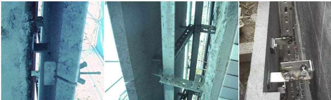
Figure 2. Attachment device types of exterior stone veneers.
