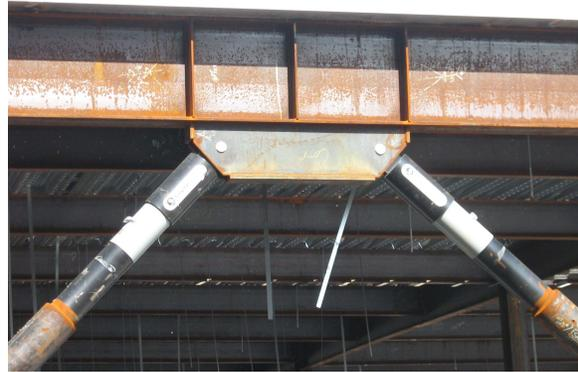
Figure 1. Viscous dampers used for design of a new building in California
