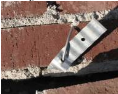
Figure 11. Deformed Anchor
