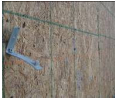
Figure 9. Anchor Pullout
