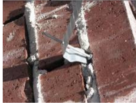
Figure 7. Typical Nail Extraction
