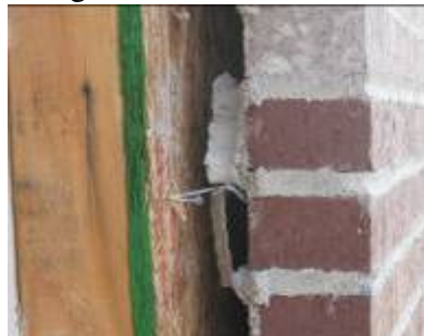
Figure 12. Anchor Extraction
